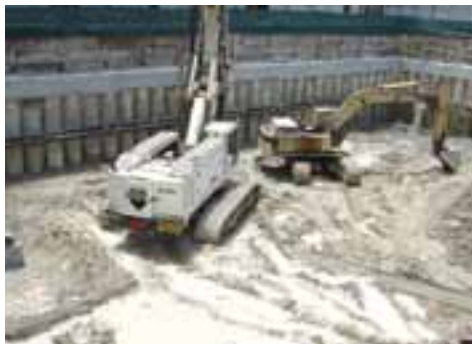
Foundation Contracting and Enabling Work - Saile Foundation LLC
